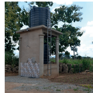
The mechanised borehole, tank and dispensing platform for East Dobro
